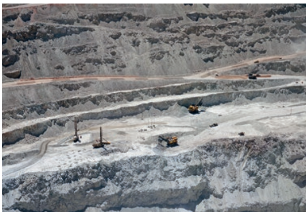
The Chuquibambilla open pit copper mine is the biggest of its kind and located in one of the driest places in the world – the Atacama Desert in Chile.
